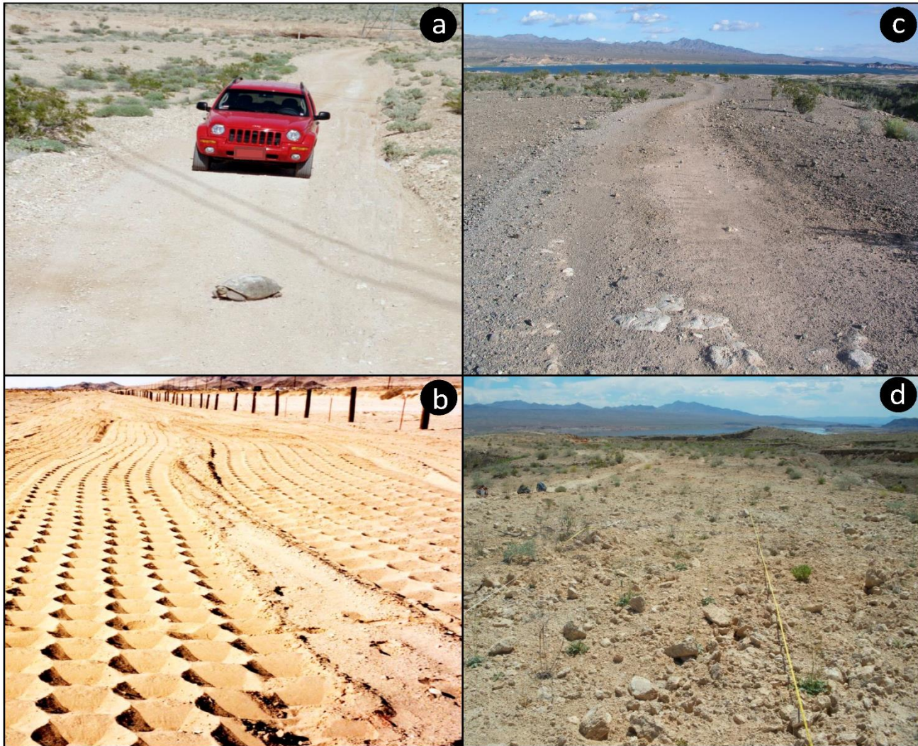
Fig. 2. Backcountry roads do pose risk to desert tortoises (a). Imprinting (b) to enhance water retention and plant establishment on a decommissioned road. Ripping road surfaces (d), compared to no ripping (c), can roughen compacted soil and promote plant recruitment. Photo credits: a) R.J. Abella; b) D.A. Bainbridge; and c,d) S.R. Abella.
