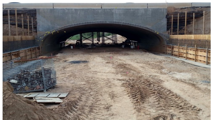
Oracle Road Wildlife Underpass under construction in September 2015. Photo by Coalition for Sonoran Desert Protection.
