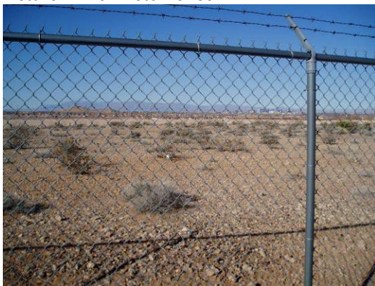
Picture D: Perimeter fence
